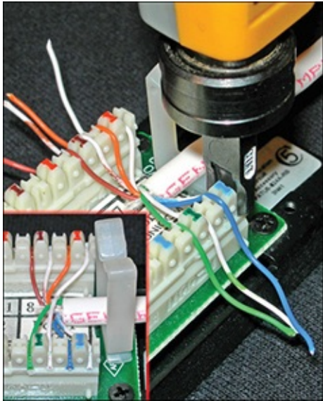
FIGURE 6.18 Punchdown tool inserting wires into an IDC
